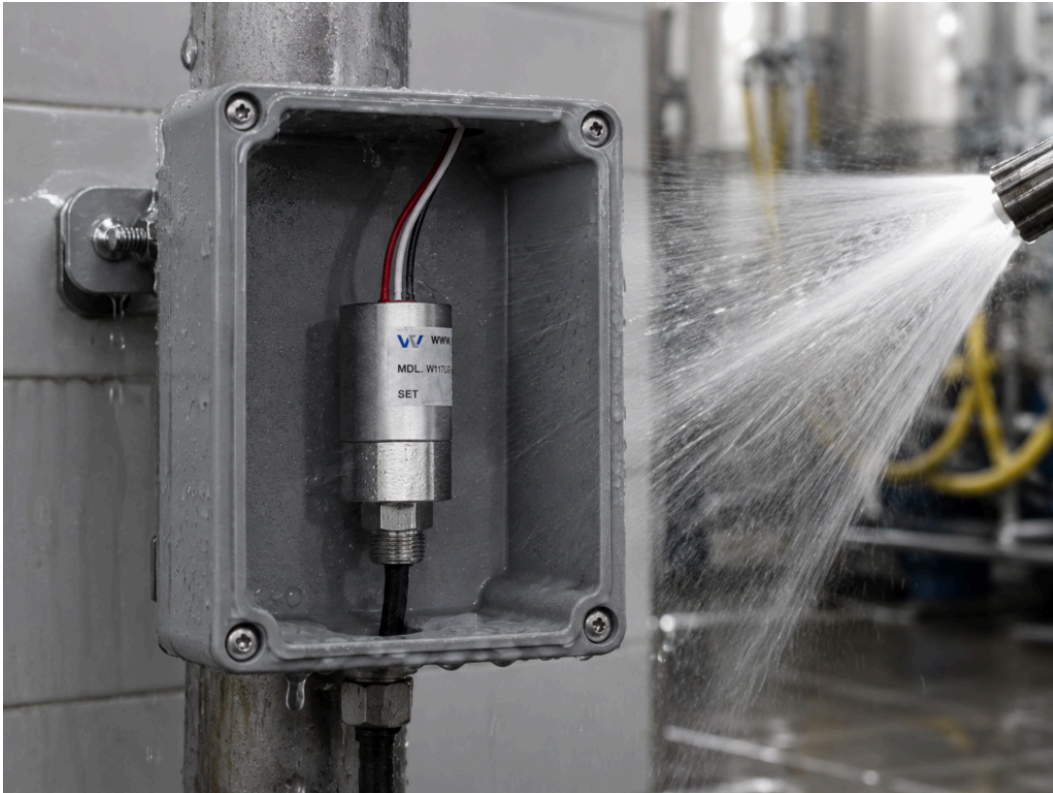
A sealed enclosure or junction box being sprayed with a hose in a washdown area.
